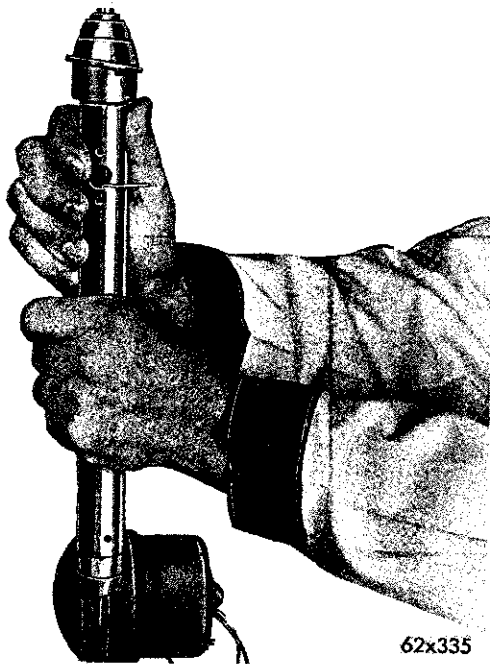
Fig. 7—Installing Mast Support
