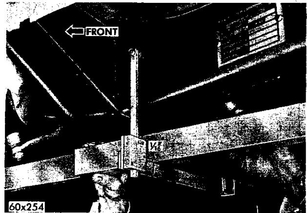
Fig. 16—Checking Body to Frame Alignment
