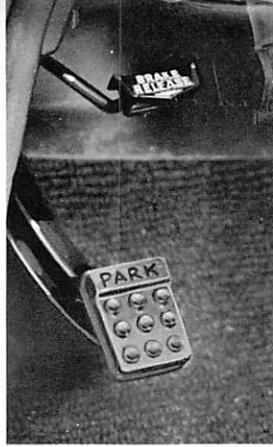
New convenience and ease of operation are provided for Chrysler's independent parking brake. Just step on the pedal, located at the left side of the cowl, and the parking brake is set. To release it, flick the release lever above it with a finger.
